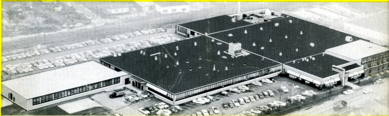
SALES, APPLICATIONS, AND TUBE MANUFACTURING FACILITY, HICKSVILLE, L. I., NEW YORK
