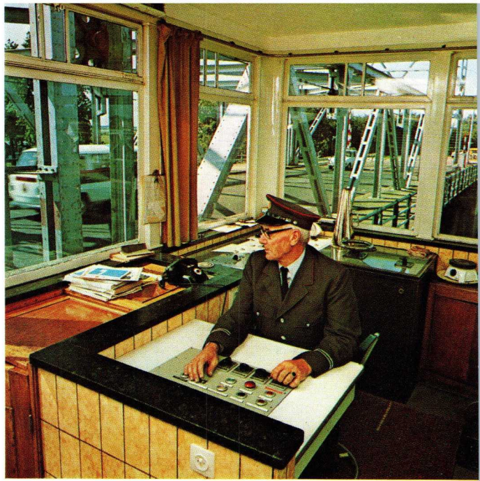
Central control desk (upper picture) and draw bridge drive motor (lower picture). Courtesy of Elektrotechnisch Bureau Langezaal & Inniger, Leiden, The Netherlands.
