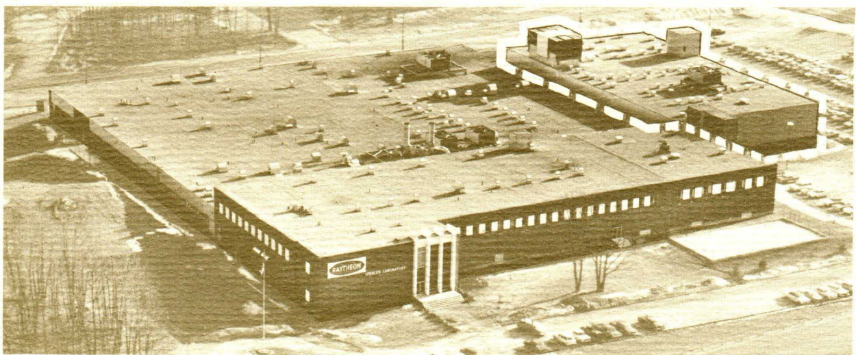
A FACILITY FOR TESTING developmental models of Super Power Amplitrons is located at Raytheon's Spencer Laboratory, Burlington, Massachusetts. The test facility occupies the 26,000-square-foot section at the upper right.
